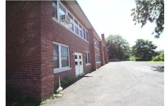
Runoff from the roof of the preschool currently drains onto pavement behind the building. The lawn area at the front can be converted into two rain gardens to capture and infiltrate this roof runoff. Downspouts may be redirected into rain barrels as well to harvest rainwater that could be used to water existing gardens behind the school. A preliminary soil assessment suggests that soils have suitable drainage characteristics for green infrastructure.
