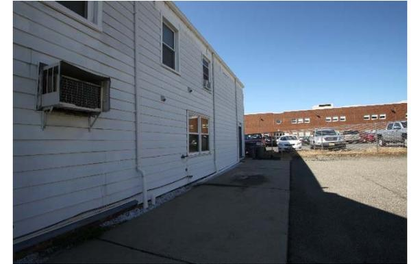
Runoff from the parking lot is currently directed towards an adjacent southeast building. Parking spots can be replaced with porous asphalt to capture and infiltrate this runoff. A preliminary soil assessment suggests that soils have suitable drainage characteristics for green infrastructure.
