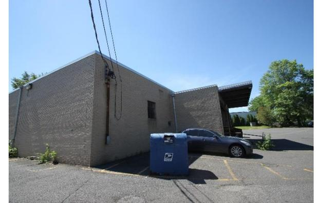
Water from the parking lot currently drains into catch basins behind the building. Parking spots can be replaced with porous asphalt to infiltrate this runoff. Downspouts can also be disconnected into a rainwater harvesting system as well. A preliminary soil assessment suggests that more soil testing would be required before determining soil suitability for green infrastructure.
