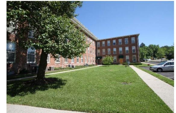
Runoff currently flows into catch basins within the parking lot or pools in lawn areas next to the building. Parking spaces can be replaced with porous pavement to infiltrate runoff from the parking lot. Rain gardens can also be planted between the building and parking lot, to capture, treat and infiltrate roof runoff. A preliminary soil assessment suggests that soils have suitable drainage characteristics for green infrastructure.
